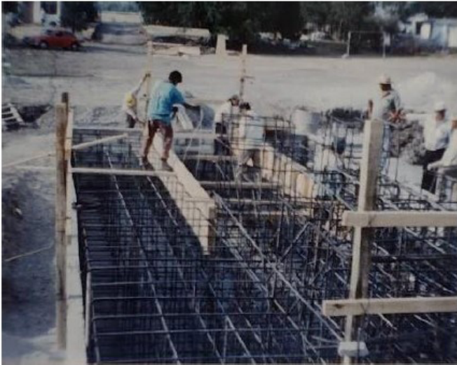
Figure 5. Reinforcing Steel in the foundation block
