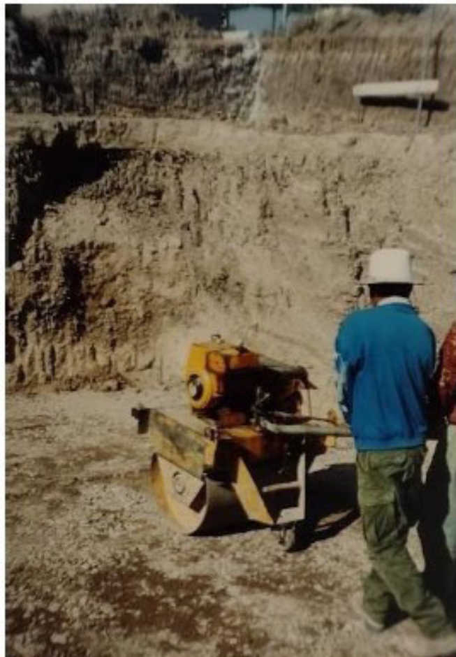
Figure 4. Compaction of the base layer (gravel - sand)
