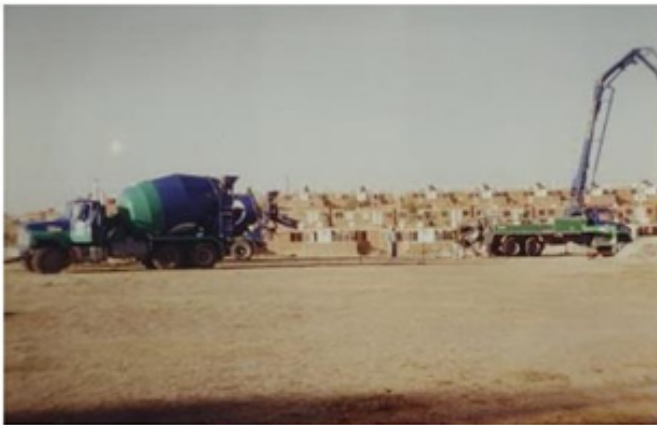
Figure 6. Casting of the foundation block
