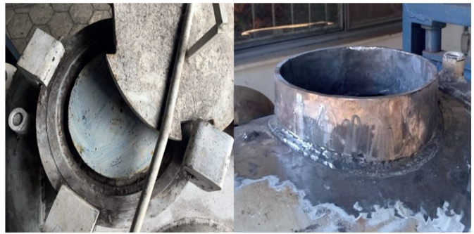
Figure 5. Old hyperbaric chamber hatch (left), Upper access opening resulting from flange removal (right).
