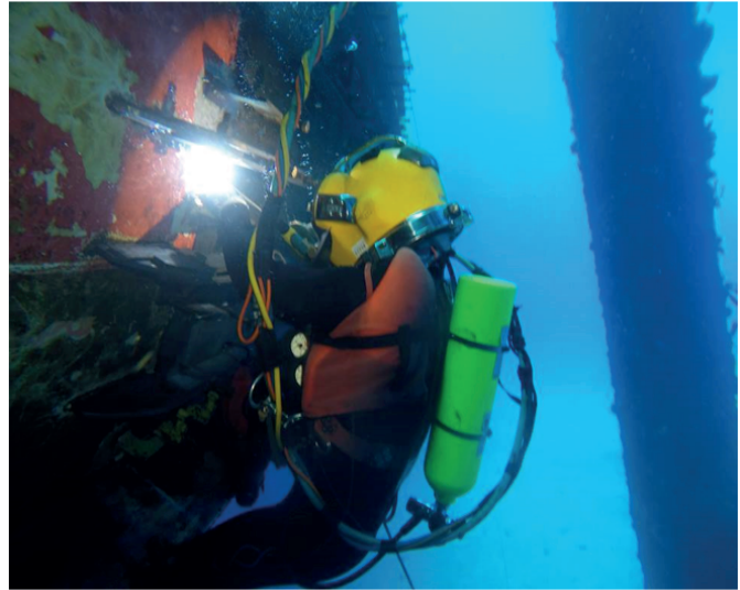
Figure 1. Welder performing the underwater wet welding process [4].
